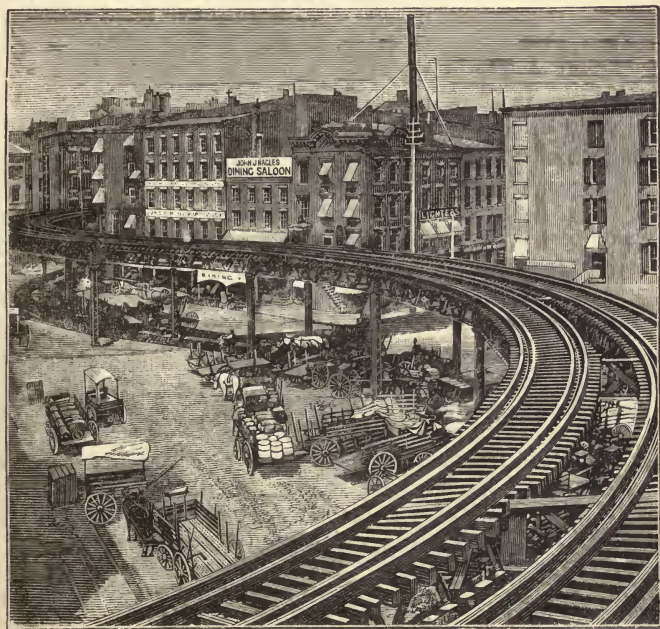
THE ELEVATED RAILWAY.
